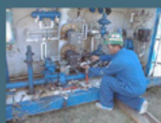
Gas Production Monitoring
