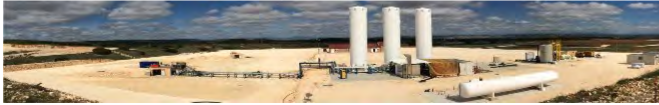
Hontomin , Spain: unique onshore pilot CO 2 injection site in the EU , recognized by the European Parliament as a key test facility (E.P. Resolution 2014) Deep saline aquifer – carbonates – 1500 m depth
