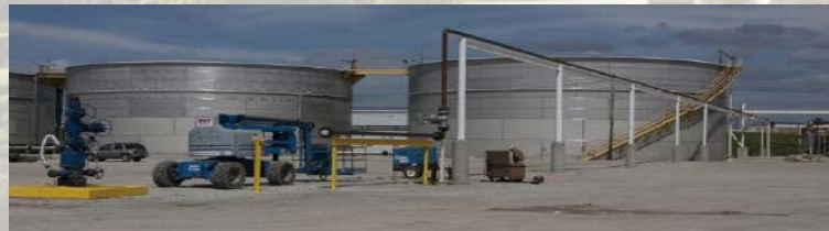
CO 2 Pipe to Injection Well
